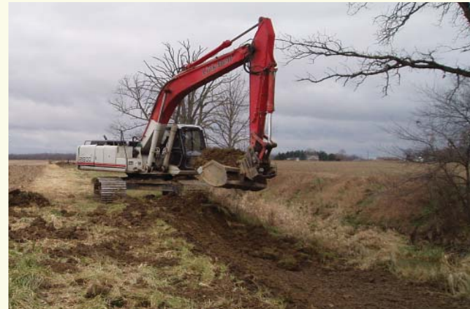
During construction 11,565 cubic yards of material was removed.
