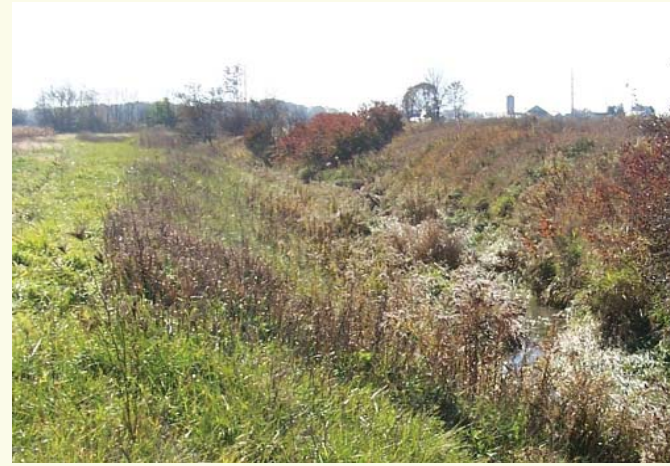
Klase Ditch prior to redesign. Note the v-shaped channel.
