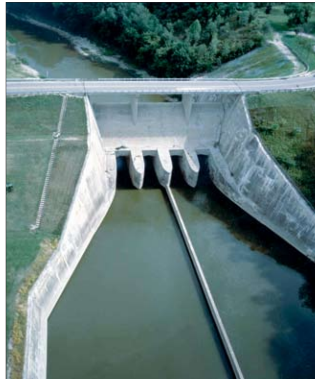
Taylorsville Dam near Vandalia is one of MCD's five flood-protection dams.
